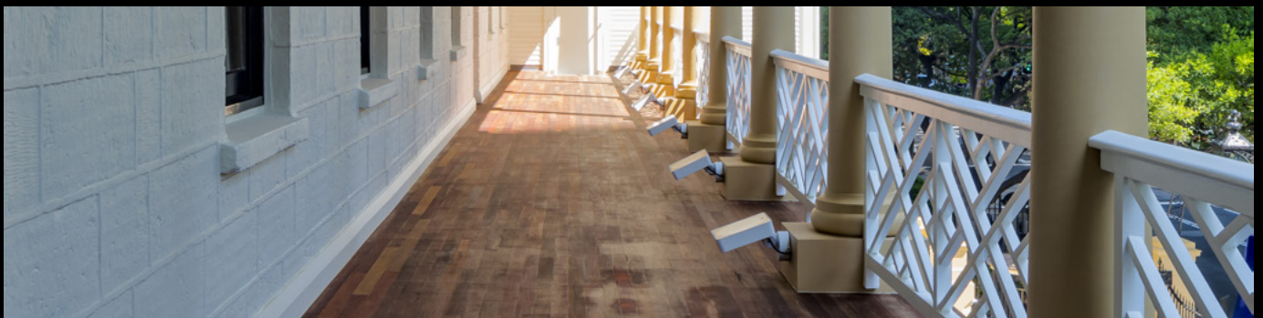
Recycled power poles.
